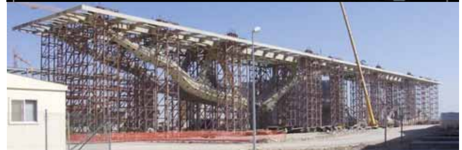
Polygonal inner constructive modules covered with external metal sheets bended accordingly ( http://www.beta.iloveqatar.net )
