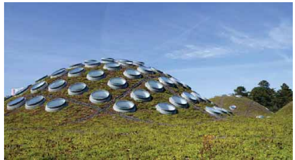
Sky lights lightens the interior garden with natural light
