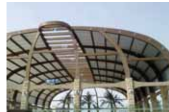
Technion pool wood structure
