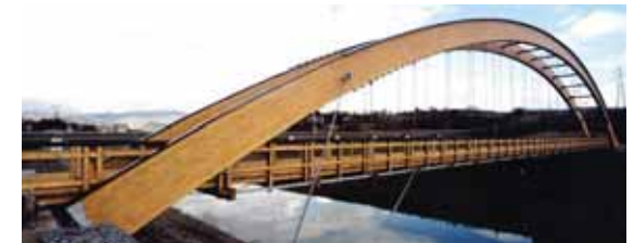
Bonatti Bridge – Firenze. Length - 76m http://www.habitatlegno.it/en/wood-accomplishments/bonatti-bridge/
