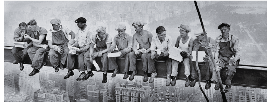
( www.dailymail.co.uk ) Eleven workmen in New York sit and eat lunch on this beam in 1932
