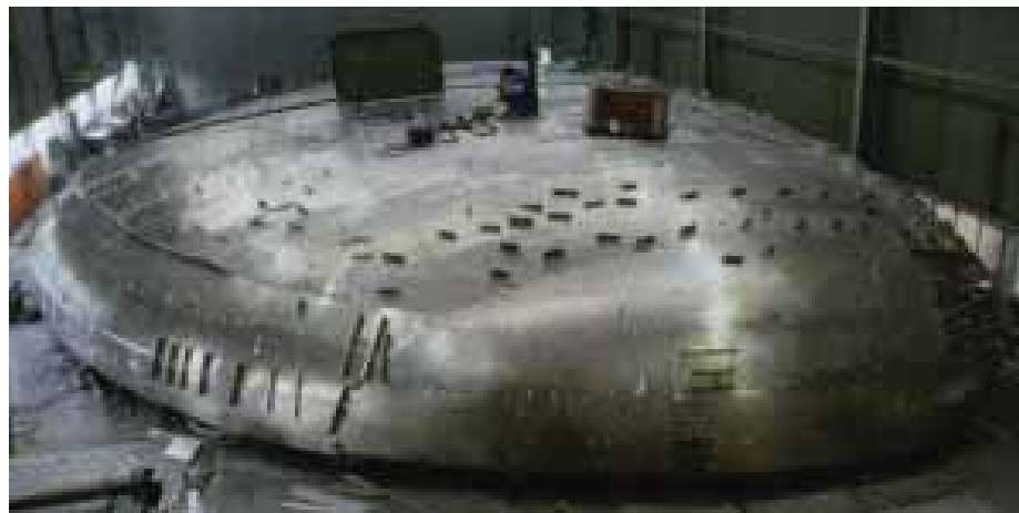
Semi Monocoque aluminium building - constructed in a boatyard ( http://www.mimoa.eu )
