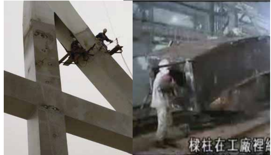
The modules being weld to another
